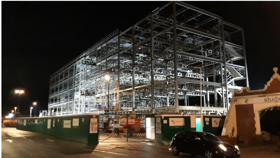
Teville Gate House Construction 12/12/2019
